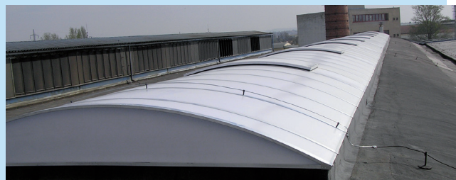
New skylights above the 3rd hall of the foundry
